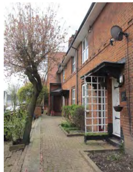
Elevated forecourt on Norton Gardens
