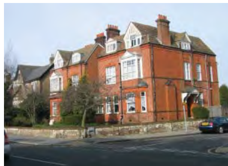
Numbers 179-183 Lower Addiscombe Road, within the Inglis Road LASC
