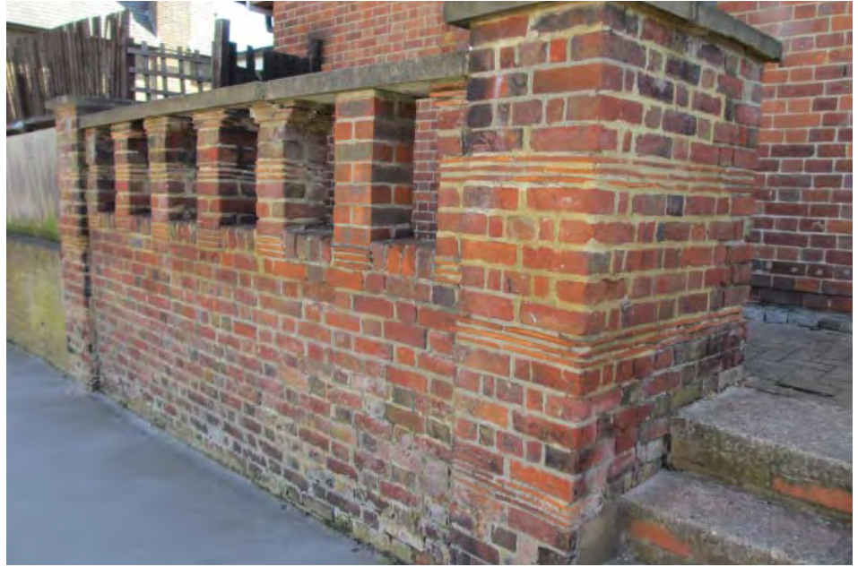
Original brick boundary treatment with clay tile slips
