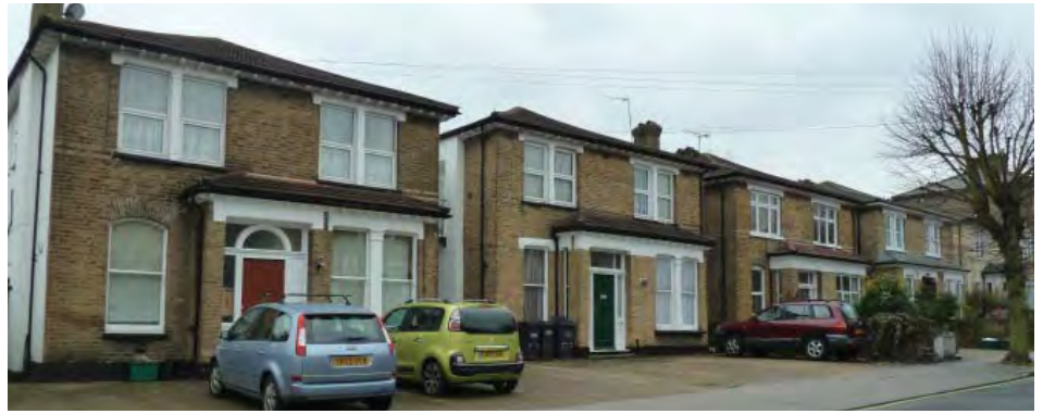
Loss of front gardens to properties on Clyde Road, leaving a stark and harsh appearance and negative impact on the streetscene
