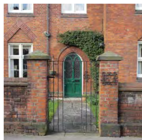
Historic entrance piers and doorway to 89 Outram Road
