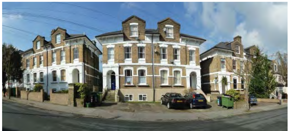
Typical sequence of three storey pairs of semis on Outram Road
