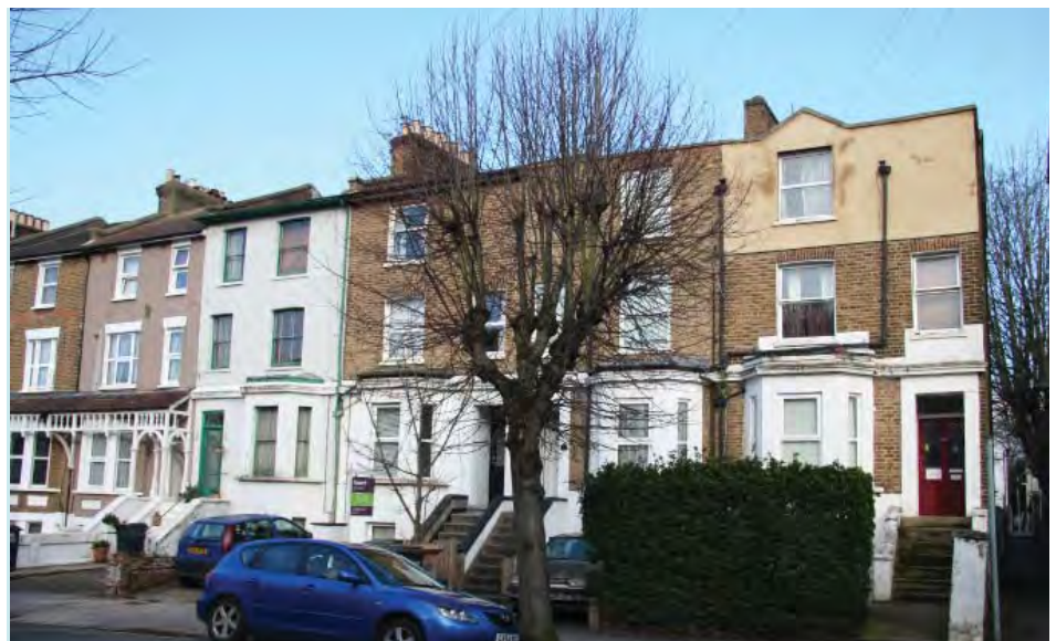
Examples of render / cladding. Not acceptable
