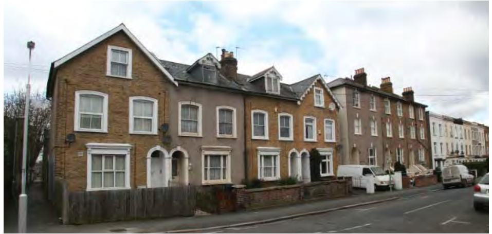
Terraces at the north of Elgin Road
