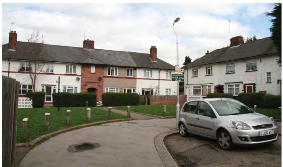
Square opening onto Northborough Road
