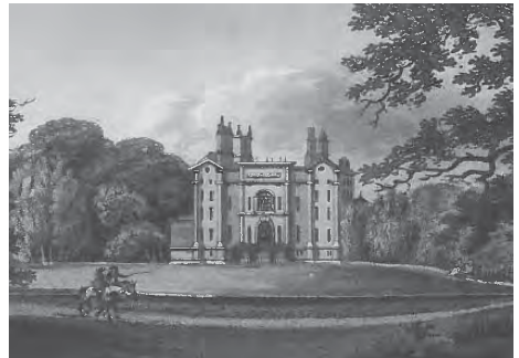
18th century etching of Addiscombe House
