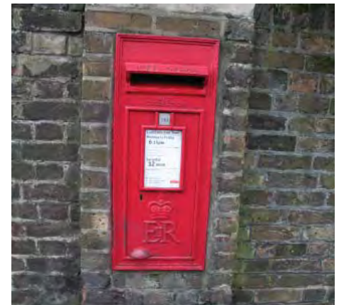
Cast iron wall mounted post box on Lower Addiscombe Road
