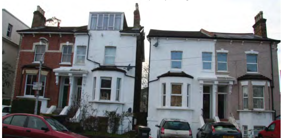
Photograph illustrating a range of alterations that have harmed the appearance of two pairs of semi-detached buildings, including an oversized dormer, render and pebbledash application, uPVC windows, the loss of a chimney stack and car parking where there would have once been a front garden
