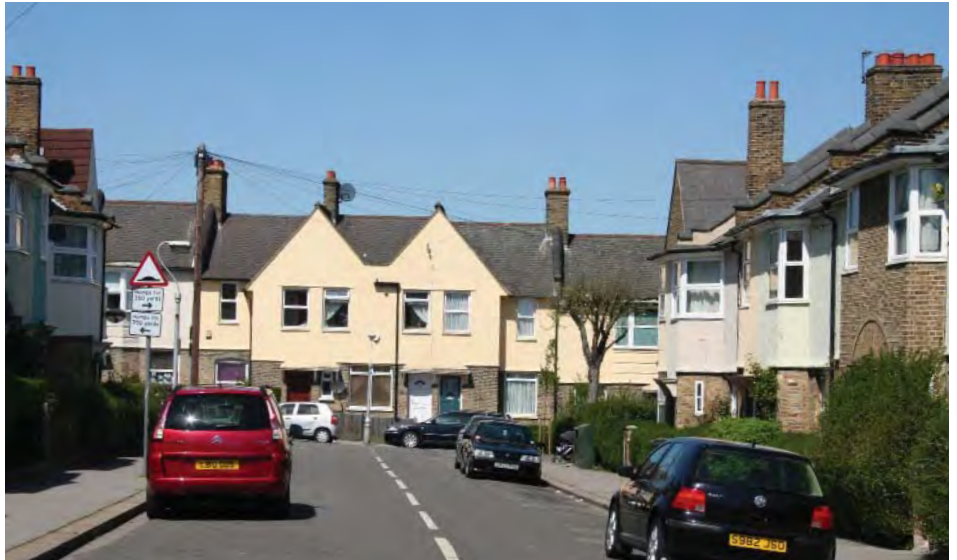
View north on Granden Road from the crossroads with Newlands Road with the closed vista of a double gable in a terrace on the north side of Northborough Road
