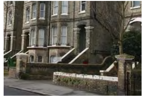
Low walling boundary treatment with brick piers topped with stone coping
