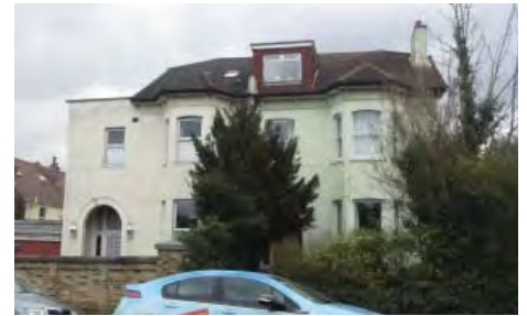
Poor quality extensions to a building on Havelock Road - the side extension is not set back from the front wall of the house and does not respect the building's character and design and the roof extension is oversized and of an insensitive design.
