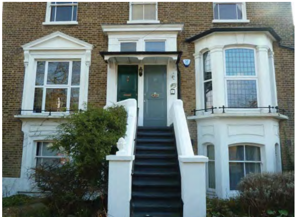
An examples where a property conversions has distorted the original symmetry of the building by creating an additional doorway
