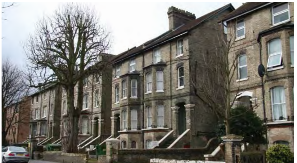
Numbers 23-28 Canning Road, an important grouping of four pairs of three storey semi-detached buildings with raised ground floors and basements
