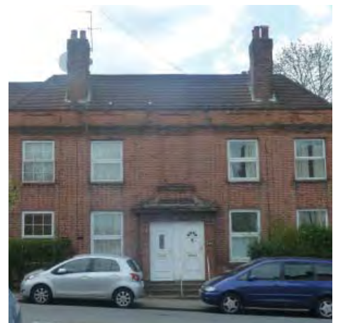
Uncoordinated window replacement that has harmed the collective character of the building
