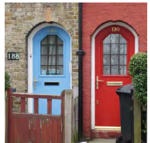
Part glazed timber doors - original design features
