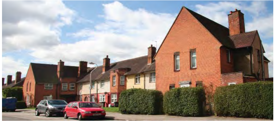
Thirteen houses forming a terrace on Isham Road. An example of street-facing gables framing both ends of the terrace.
