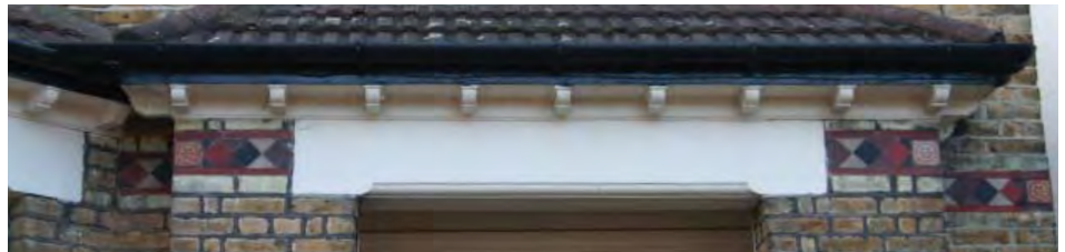
Decorative window framing at 87 Elgin Road
