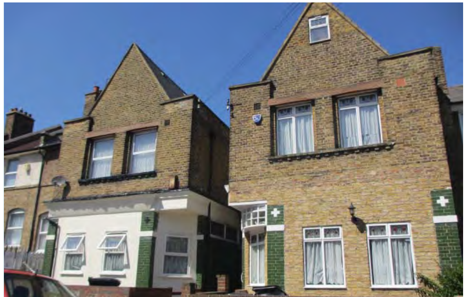
Former shops in Newlands Road (numbers 80-82) as they are today
