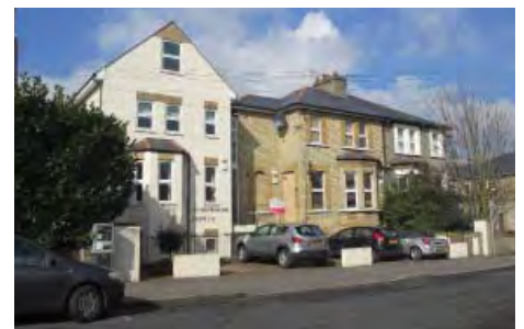
Oversized extension (left) of a poor quality design and materials
