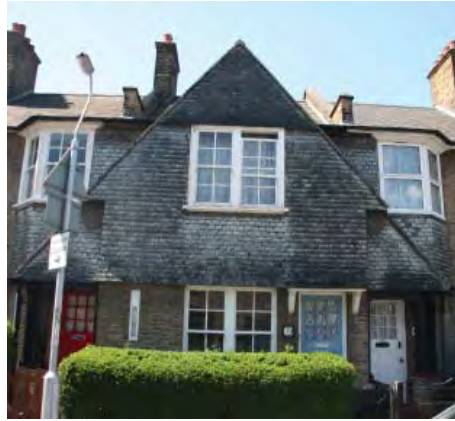
Gable containing three houses
