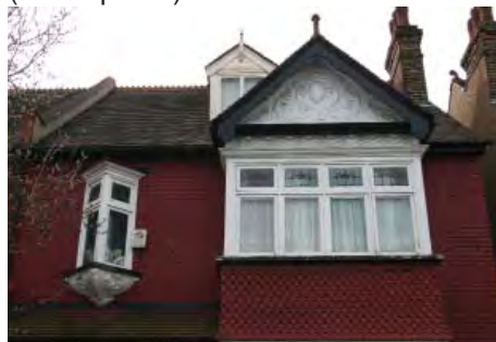
Plasterwork detailing at number 170
