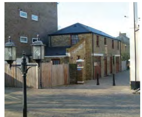
One of the historic Professor's Houses on Addiscombe Road was recently converted into flats, and the former Coach House was converted into two small houses. The work was carried out to a high quality and has resulted in an enhancement to the character and appearance of the conservation area.
