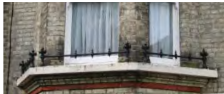
Architectural detailing of London brick elevations
