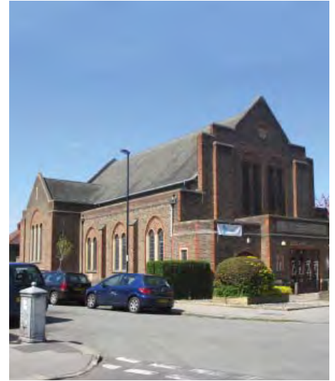
Norbury Baptist Church, located within the setting of the Norbury Estate to the north
