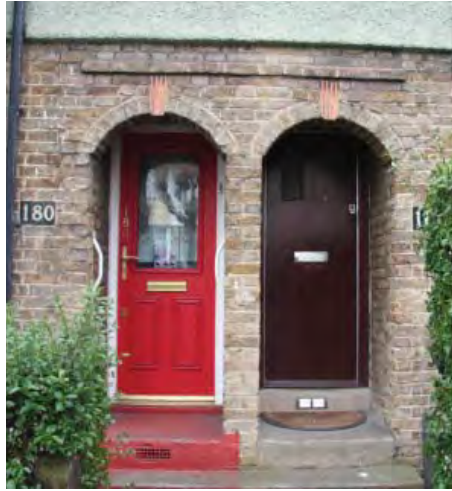
Well preserved recessed doorways
