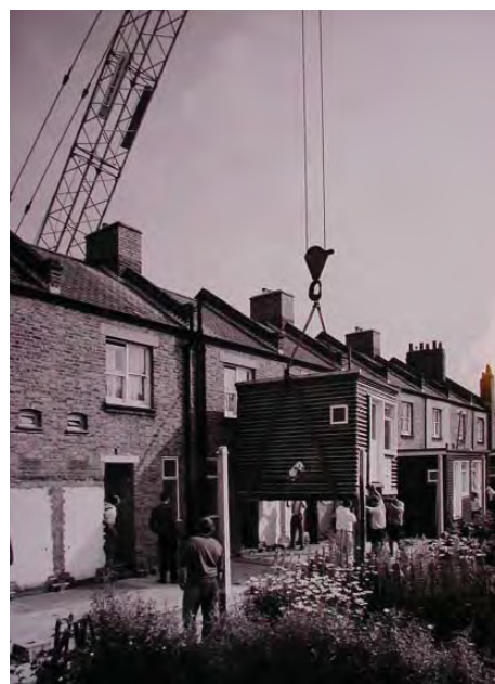
Modernisation of 1970s: rear extensions with toilet facilities
