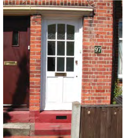
Part-glazed timber door on Tylecroft Road
