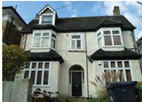
The original character of this building has been eroded by the introduction of render, the installation of uPVC windows at ground floor level and the installation of a dormer window to the front roofscape
