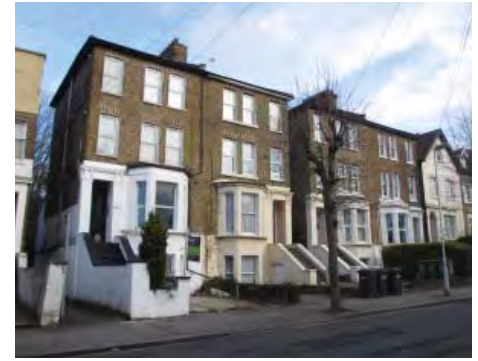
Three storey semi-detached buildings on Canning Road with additional lower ground floors
