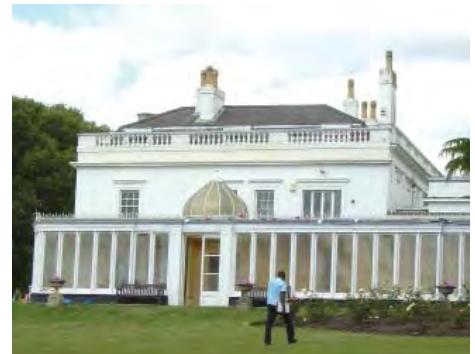
Norwood Grove Mansion from the south east showing the orangery
