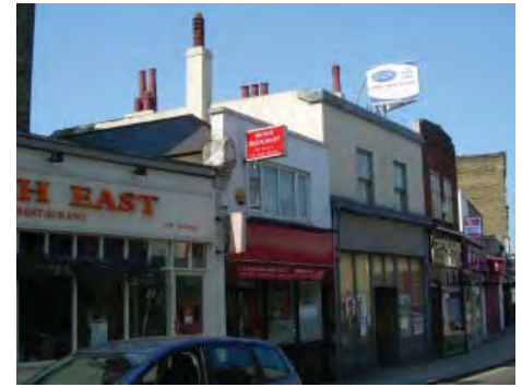
Commercial terraces on Westow Hill
