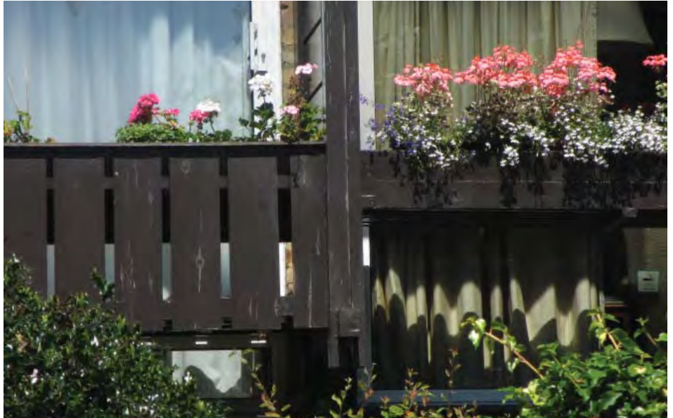
Detail of window box and balconies, important original architectural features
