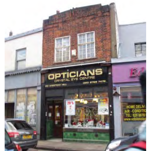
Shopfront at 20 Westow Hill (better photo needed)
