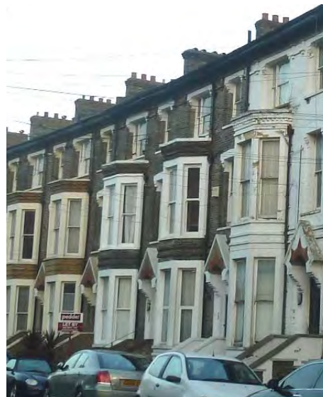
Houses on St Aubyn's Road
