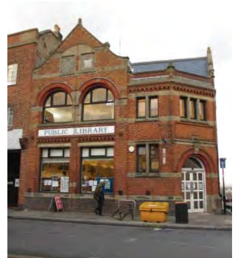
The historic Upper Norwood Library makes an important contribution to the streetscape of Westow Hill, in the direct setting of the Upper Norwood Triangle Conservation Area
