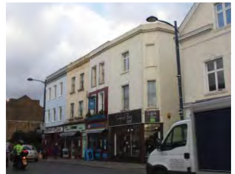
Three storey terraced buildings on Westow Street
