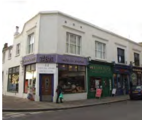
Two storey buildings on Westow Street
