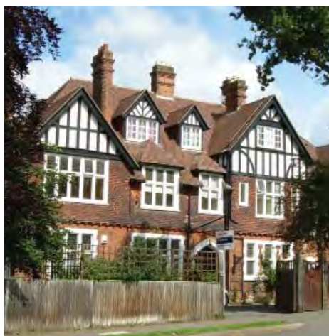
Number 69 Ryecroft Road, larger in scale and bulk than most other buildings on the road
