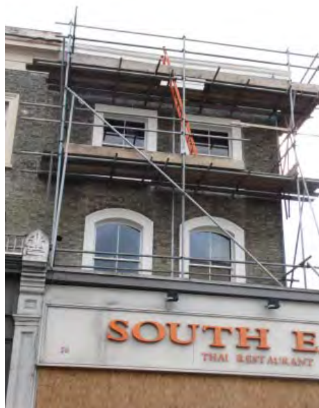
Historic features in the process of being repaired at 26 Westow Hill
