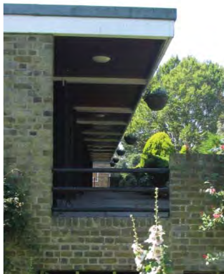
Timber overhanging canopies
