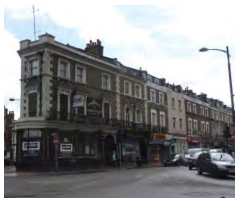
The Cambridge Pub and adjacent terrace (70-88), Westow Hill
