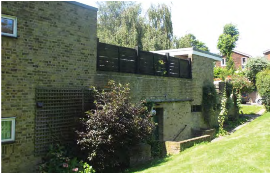
North-east end of a St Bernards terrace adjacent to the communal gardens
