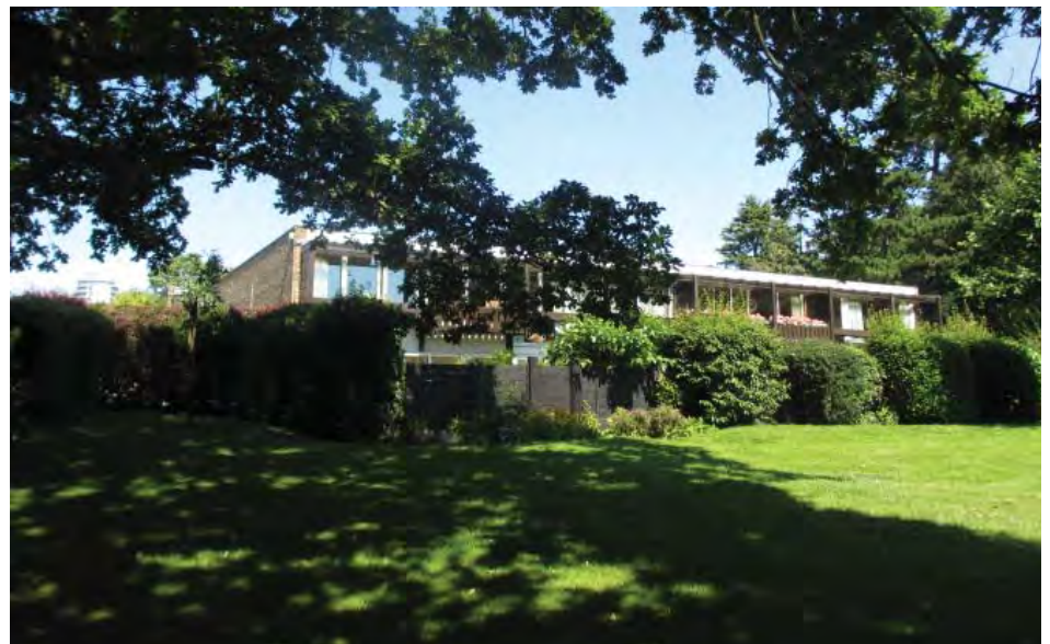
View of St Bernards from Fairfield Path
