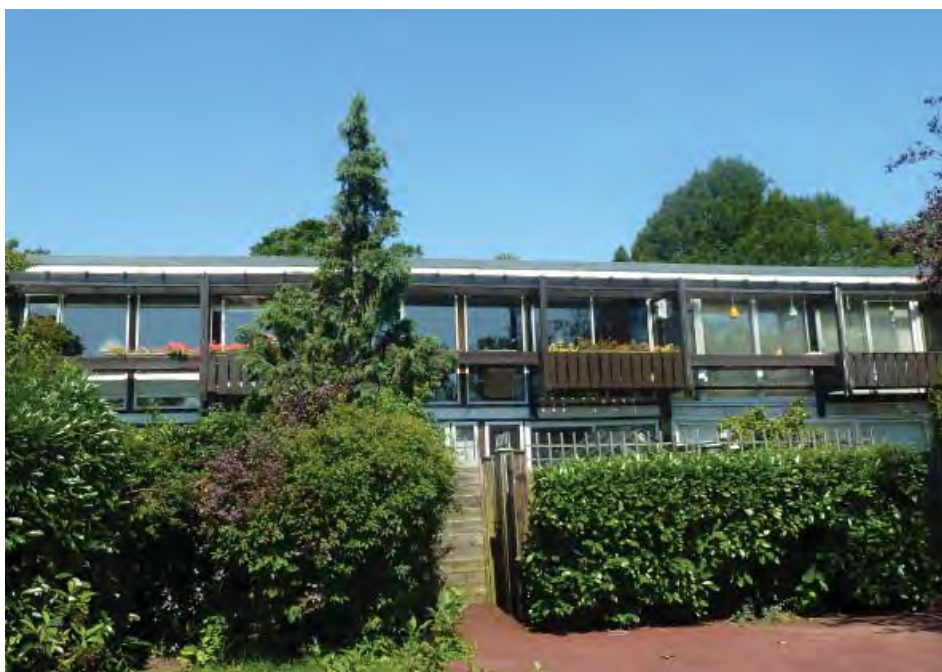
South facing elevations of a St Bernards terrace, viewed from the Piazza (see map 8 on p.15)
