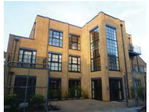
Number 6 Paddock Gardens, high quality new development that references the area's industrial character
