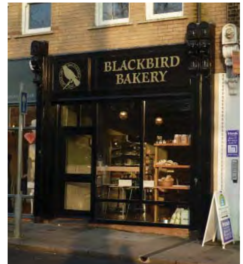
A high quality new traditional style shopfront successfully integrated within a new development on Westow Street.
