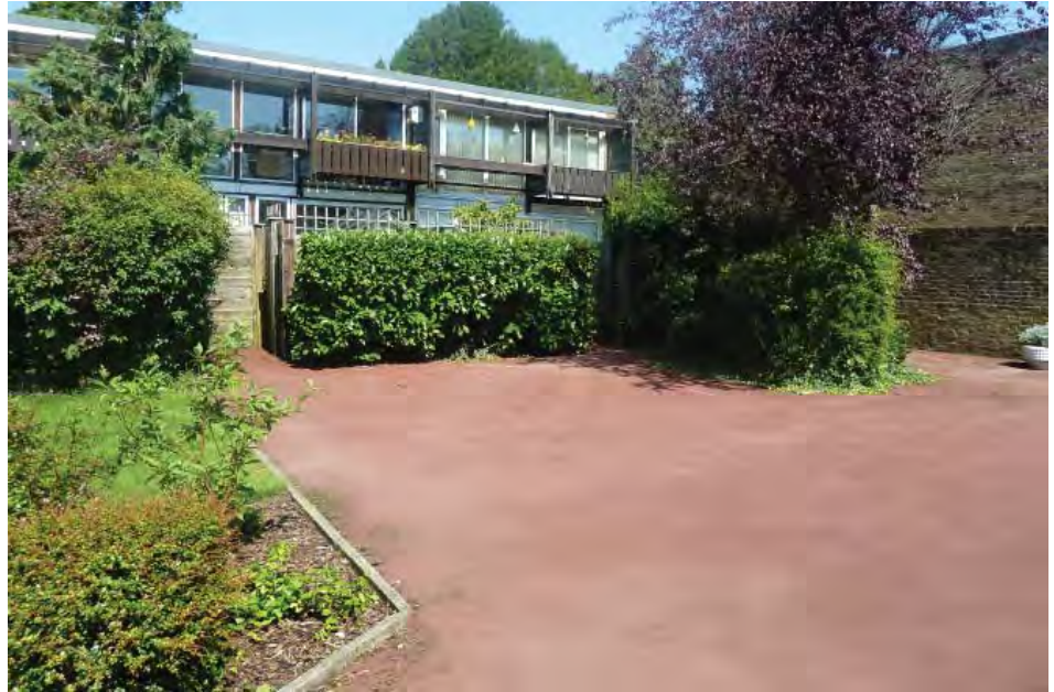
View north across the piazza towards a terrace of houses (see map 8 on p.14)
