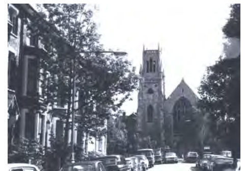
St Aubyn's Church, viewed from the north on St Aubyn's Road
