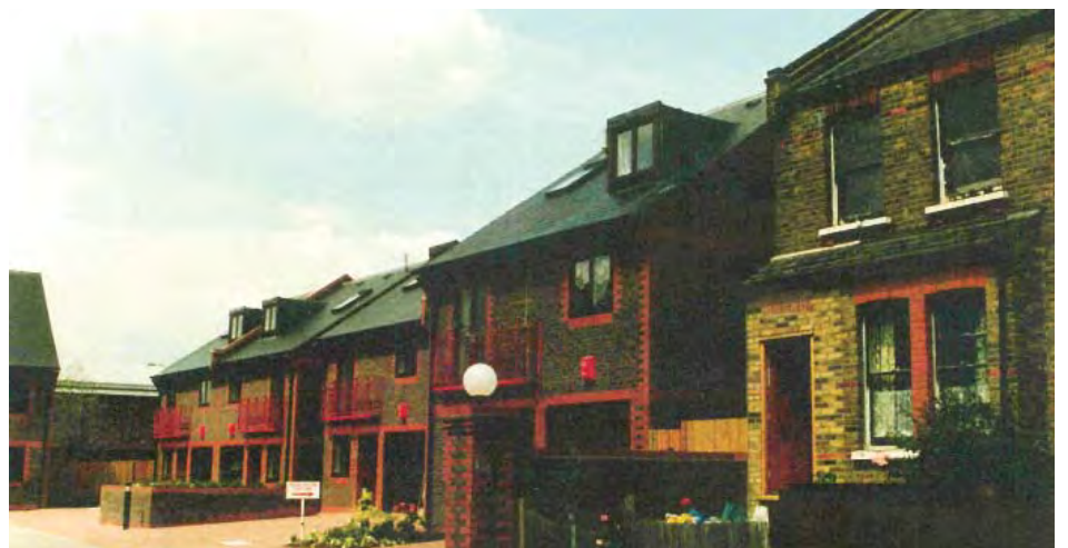
Part of the 1980s development at 16-38 Arnull's Road that replaced the demolished Victorian terraces, showing the retained number 14 to the right hand side
