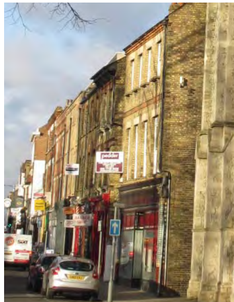
Consistent building lines along the east side of Westow Street
