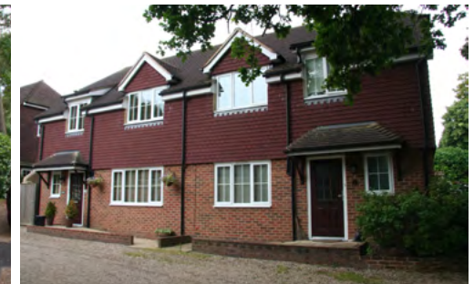
Photo 16. Compact houses on Upper Shirley Road
