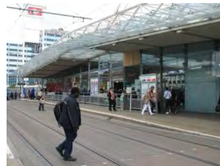
Photo 48. East Croydon Station
