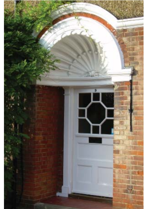
Recessed porch with intricate shell moulding and an original solid timber door in the Chatsworth Road Conservation Area
