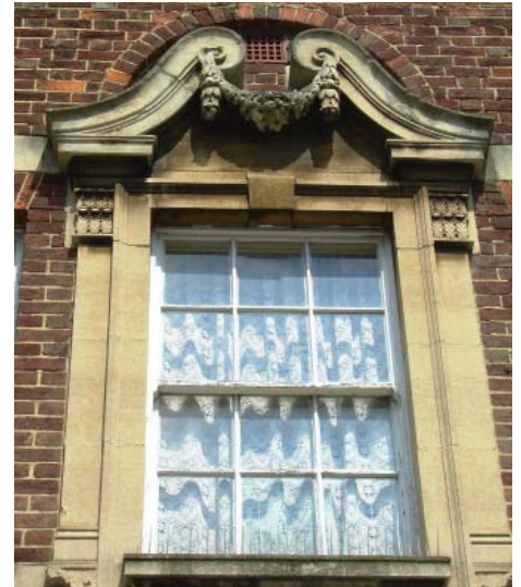
Decorative stone window surround of a timber sliding sash window in the Church Street Conservation Area. Stonework includes an architrave, pilasters and a voluted broken pediment linked by a swag.
