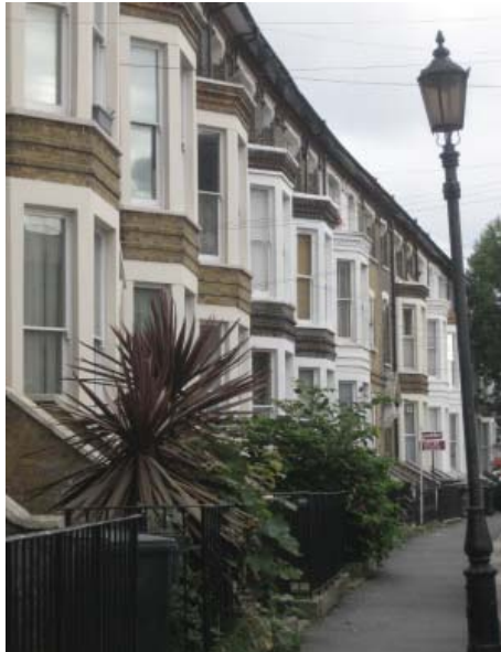
Houses on St Aubyns Road in the Upper Norwood Triangle Conservation Area, with a series of repeating bay windows
