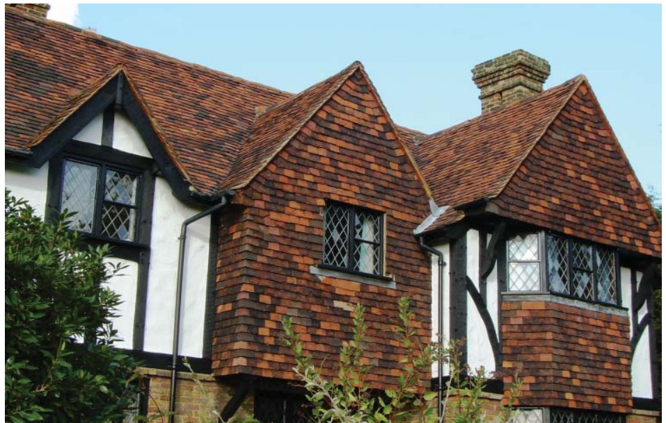
Rich materials present at a house in the Croham Manor Road Conservation Area, including hand-made clay tiles, timber facing, white render, leaded window panes and multi stock brick
