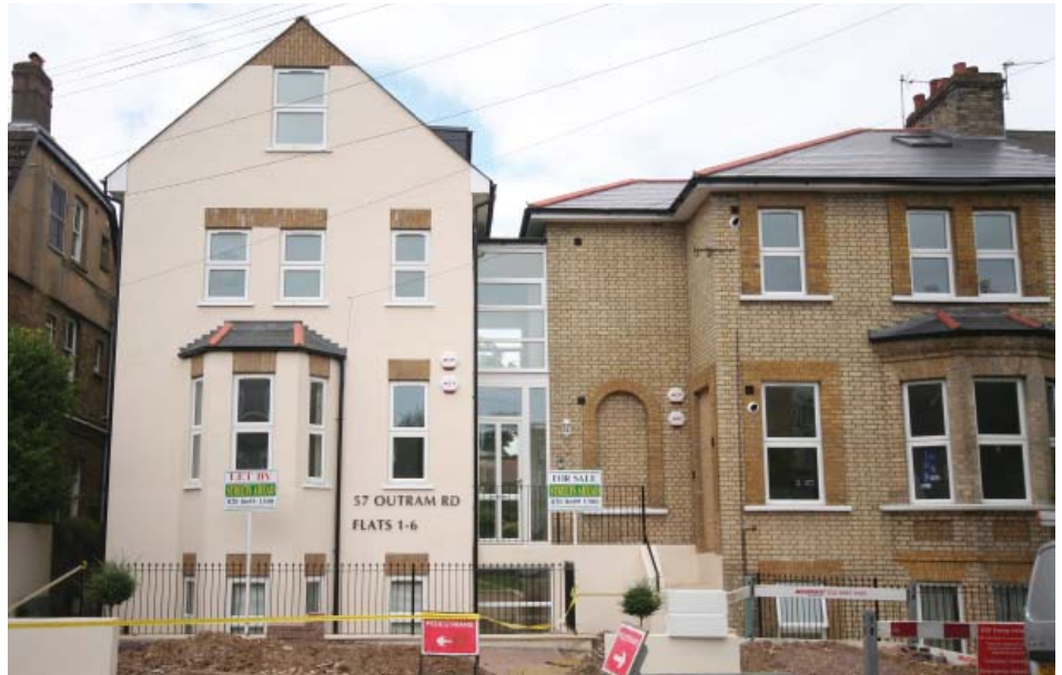
A poorly designed side extension added to a house in the East India Estate Conservation Area. The extension was designed and constructed prior to the conservation area's designation in 2008 and would not now be likely to obtain planning permission.
