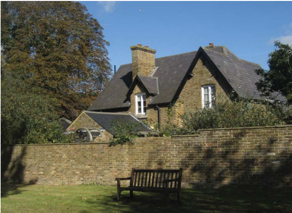
Former C19th farm cottages for Addington Park Farm in the Addington Village Conservation Area
