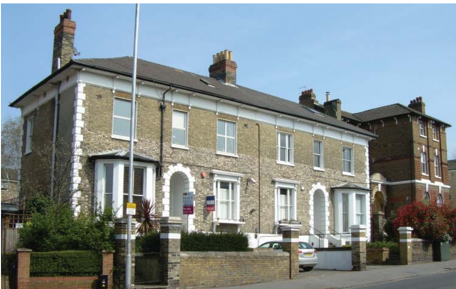
View of houses on the north side of Coombe Road
