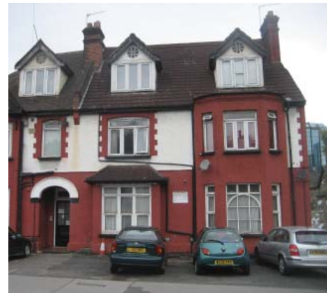
The painting of this building has resulted in harm to its character and appearance, as has the removal of a boundary treatment and introduction of hardsurfacing for car parking
