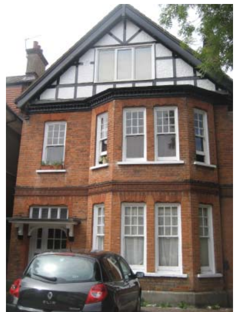
Unlisted buildings that make a positive contribution to the conservation area's special character
