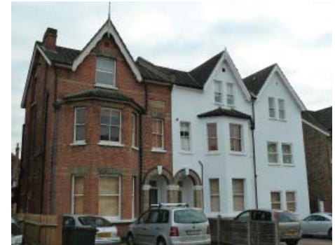
Oversized two storey extension to a semi-detached house (right)
