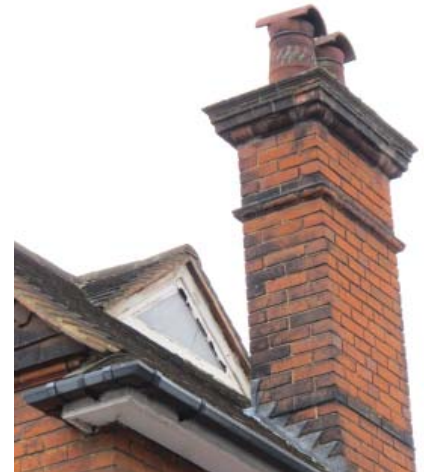
Chimney and gablet at 53 Chatsworth Road
