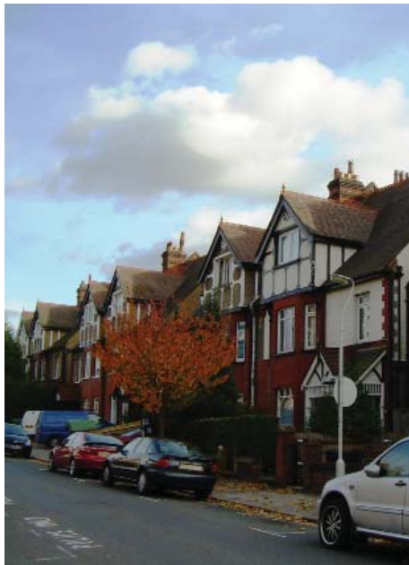
8-18 Beech House Road
