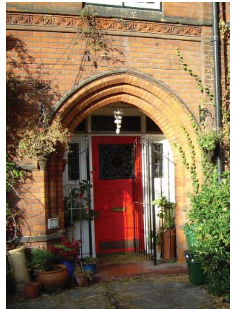
15 Beech House Road
