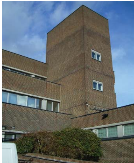
The Police Station, Beech House Road
