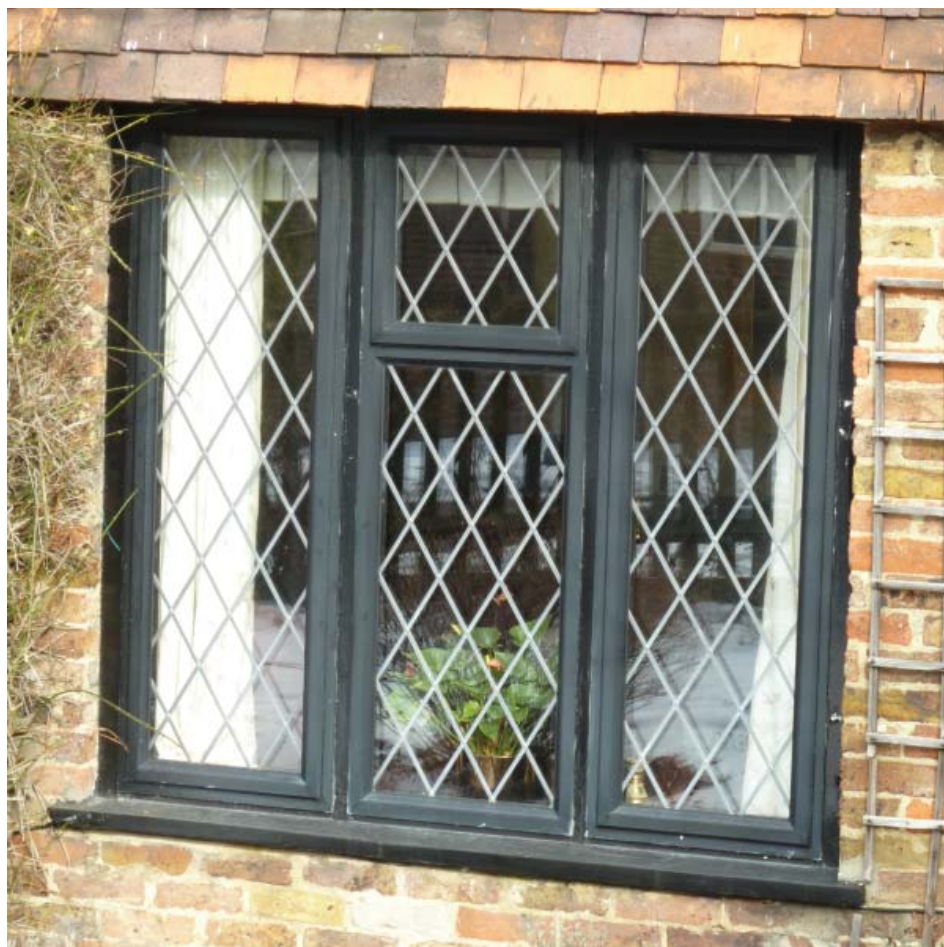
Sympathetic window replacement
