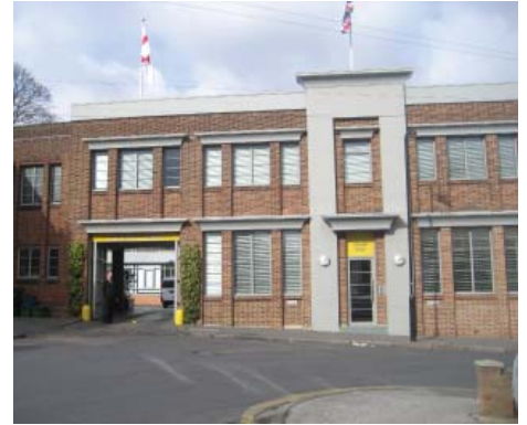
The Art Deco style entrance to 20-24 Tanfield Road (Rathbone Square)
