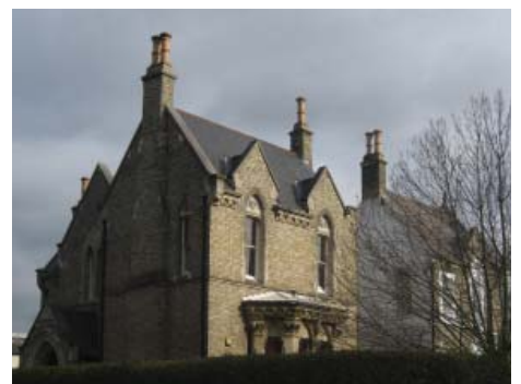
Typical building massing in the Bramley Hill character area
