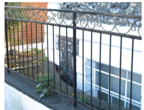
Attractive railings outside the Lodge
