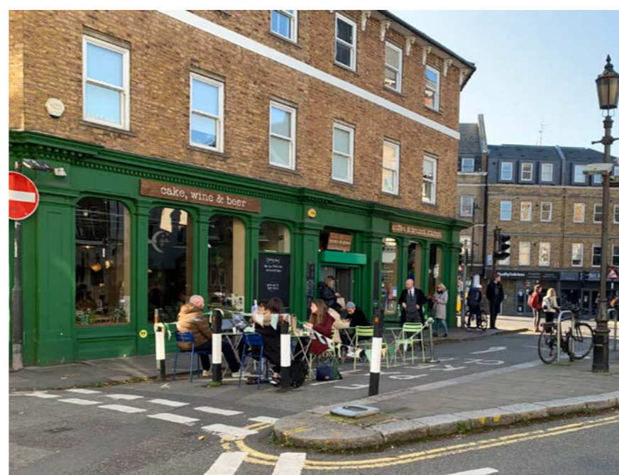
The original exit arm on Belvedere Road, now converted to an outdoor dining space
