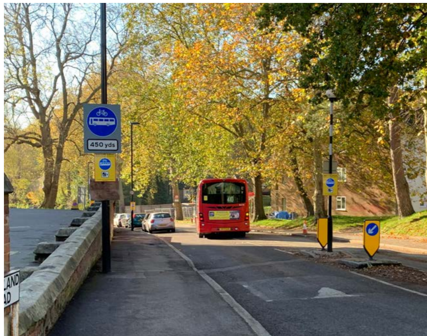
Advanced warning sign provided regarding bus gate on Auckland Road
