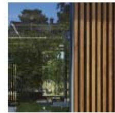
Timber fins in front of glazing to provide operable vents and solar shading
