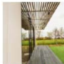
Brise soleil to teaching space external glazing
