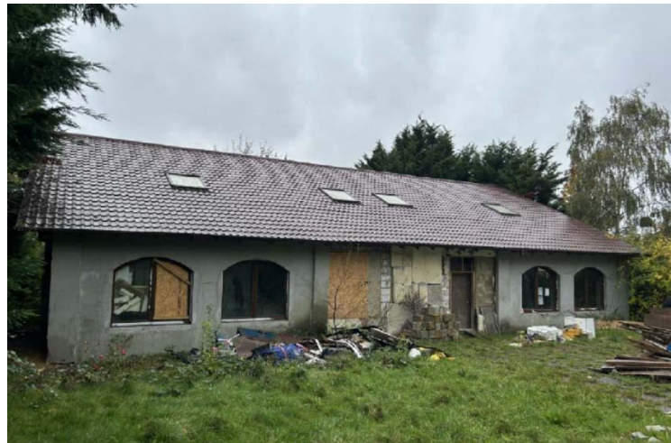
Figure 2: Photo of existing front elevation
