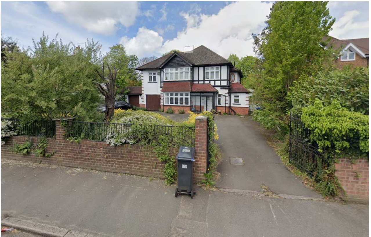
Figure 1: Street View of 172 Foxley Lane
