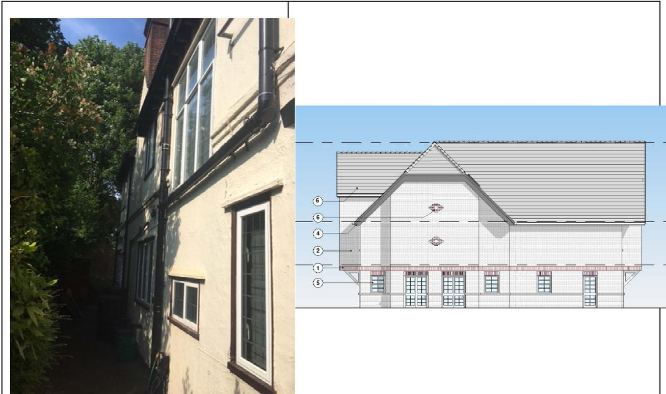
Figure 7: Existing flank elevation and proposed flank elevation
