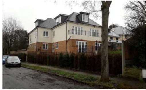
Figure4: Photograph of rear and side of site from Purley Hill
